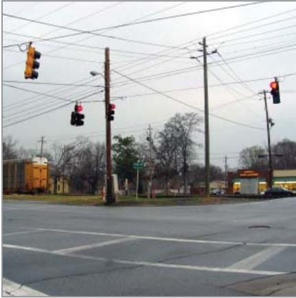
One of Hapeville's key signalized intersections is this railroad crossing at South Central and Virginia Avenues
