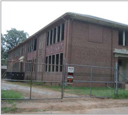
Hapeville has already started to capitalize on its historic character. The College Street School, originally Hapeville School, is undergoing conversion to lofts
