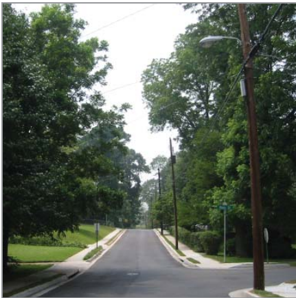
New sidewalks on North Avenue between Springhaven Avenue and Hope Street
