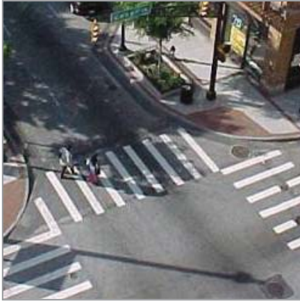
Example of Thermoplastic piano bar crosswalks
