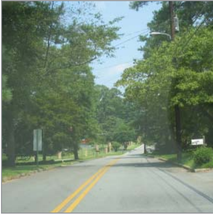
Pedestrians are forced to walk on the street in neighborhoods where there is no sidewalks on either side of the street
