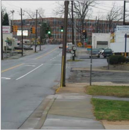
Curb cuts, utility poles and broken sidewalks create a poor public realm along this stretch of Dogwood Drive
