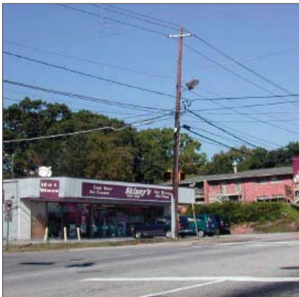
Poorly maintained crossing on Virginia Avenue (Hapeville). Average score: - 3.4
