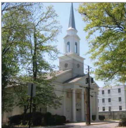
The Neoclassical style Hapeville First Baptist Church is a historic structure that must be preserved
