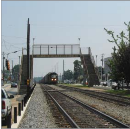
Existing pedestrian bridge over the railroad
